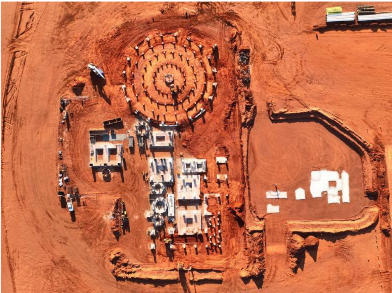
Figure 3: Thunderbird Project – Wet Concentrator Plant site concrete installation & civil earthworks
