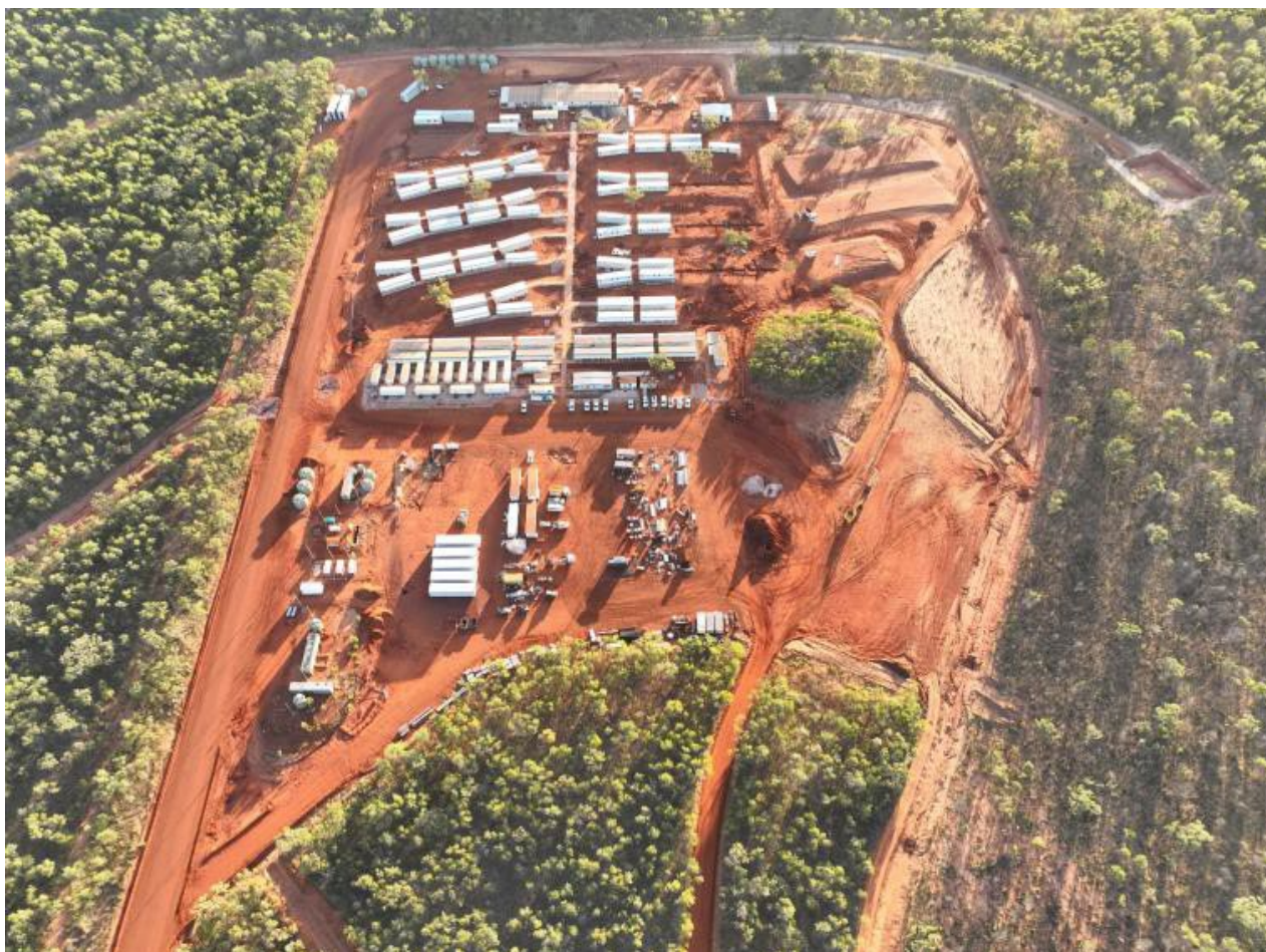
Figure 4: Thunderbird village accommodation - site works
