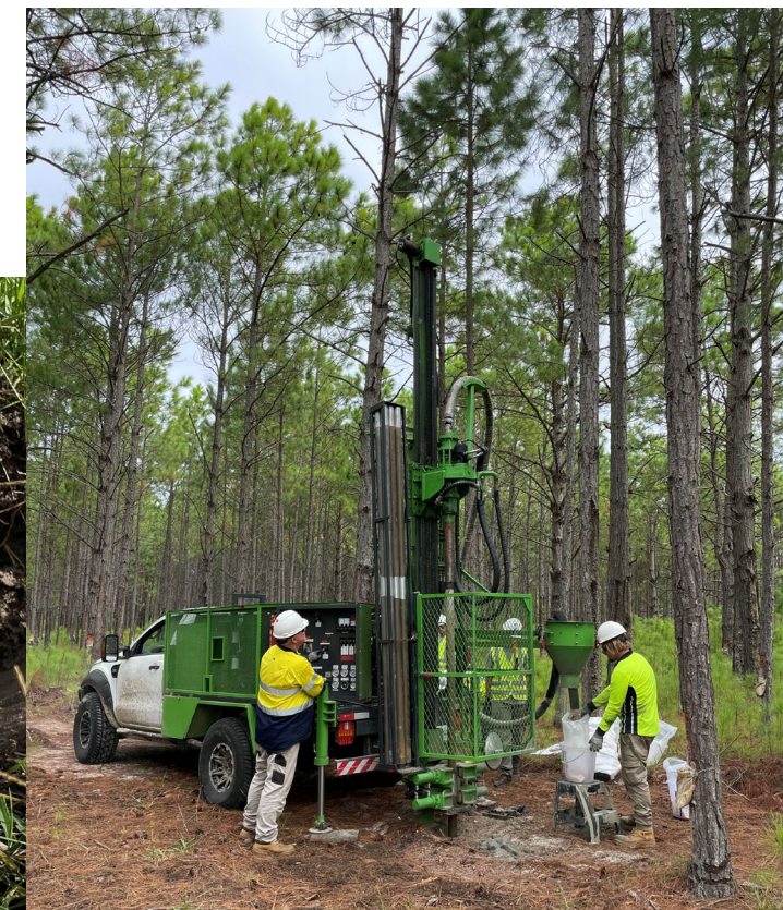
DRILLING ACTIVITIES FEBRUARY 2024
