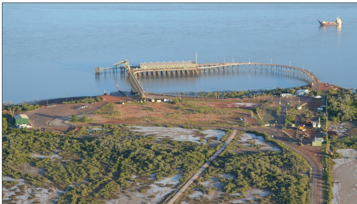
Figure 18: Port of Derby, Western Australia
