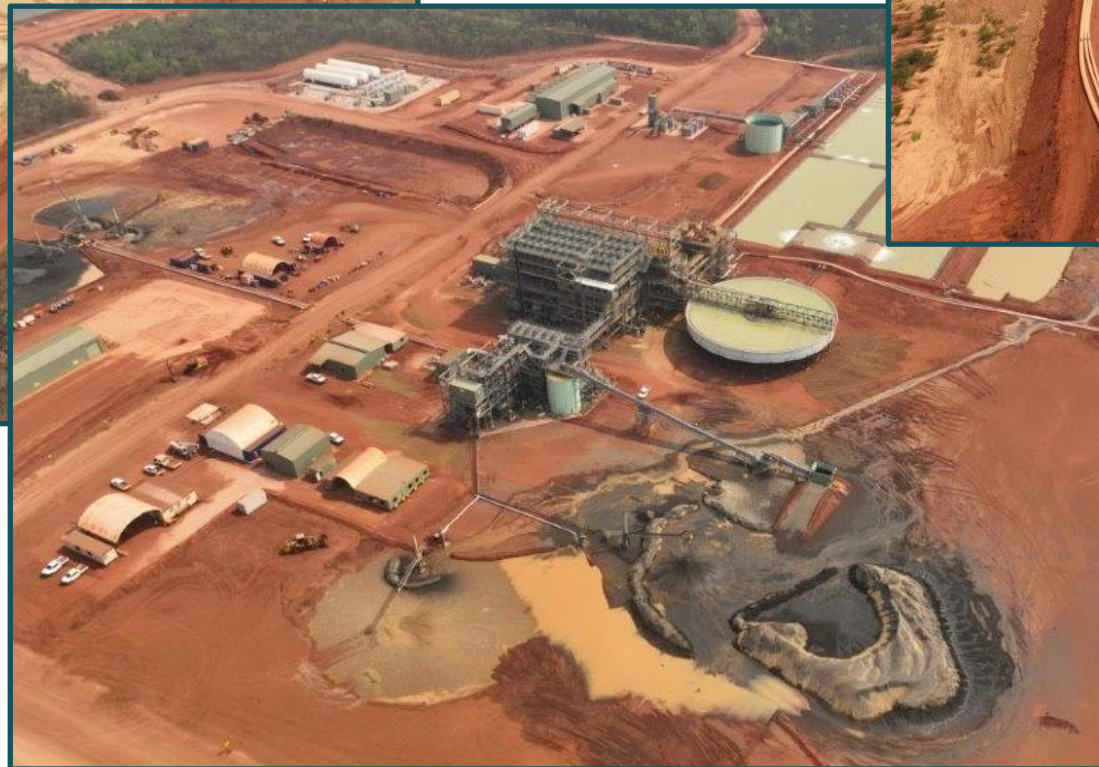
PROCESS PLANT HMC AND PRODUCT STOCKPILES NOVEMBER 2023
