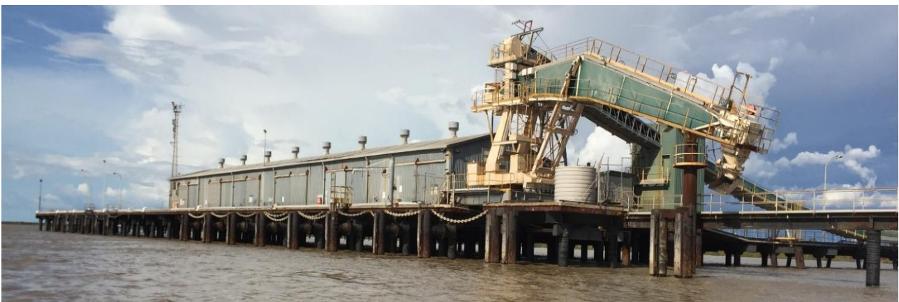
Figure 2: Derby wharf with bulk export ship loading facility
