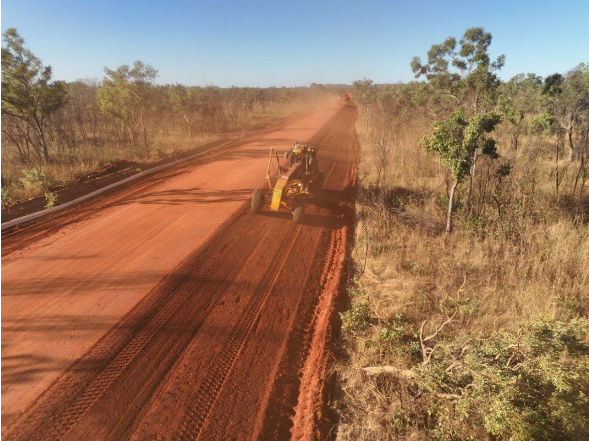
Image 7: Secondary Mine Access Road contouring
