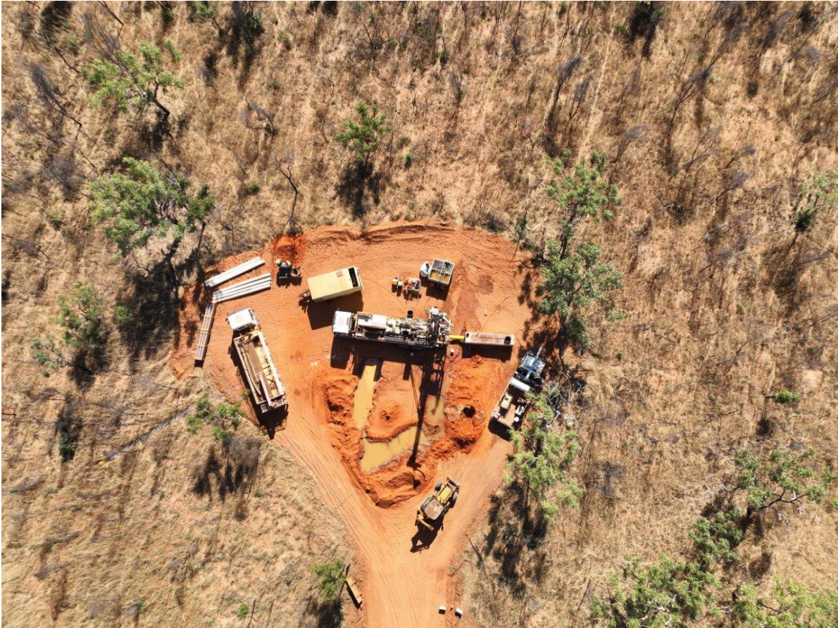
Image 3 & 4: Borefield clearing and installation activities
