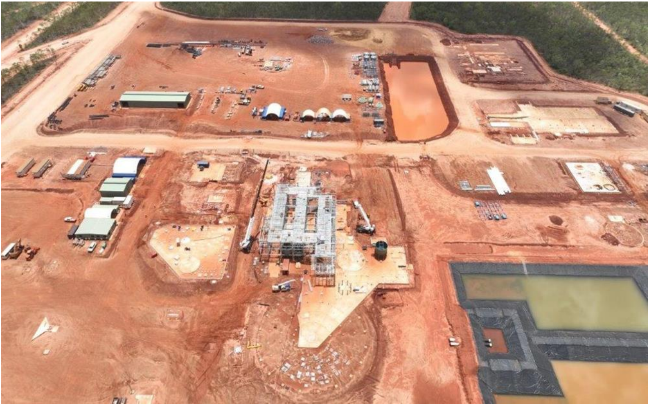
Figure 2: Process Plant Site (foreground) and laydown area (background)
