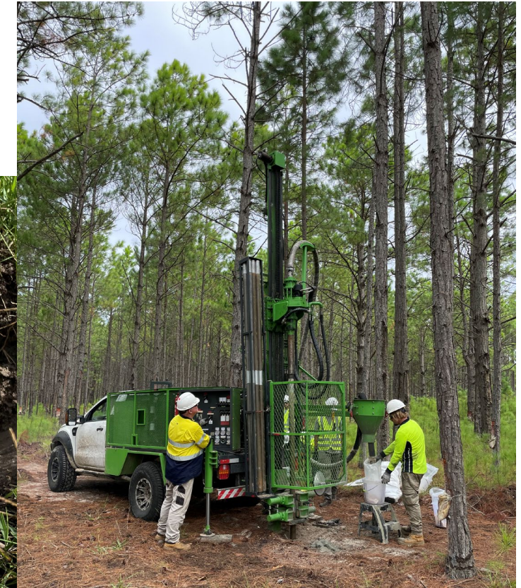
DRILLING ACTIVITIES FEBRUARY 2024
