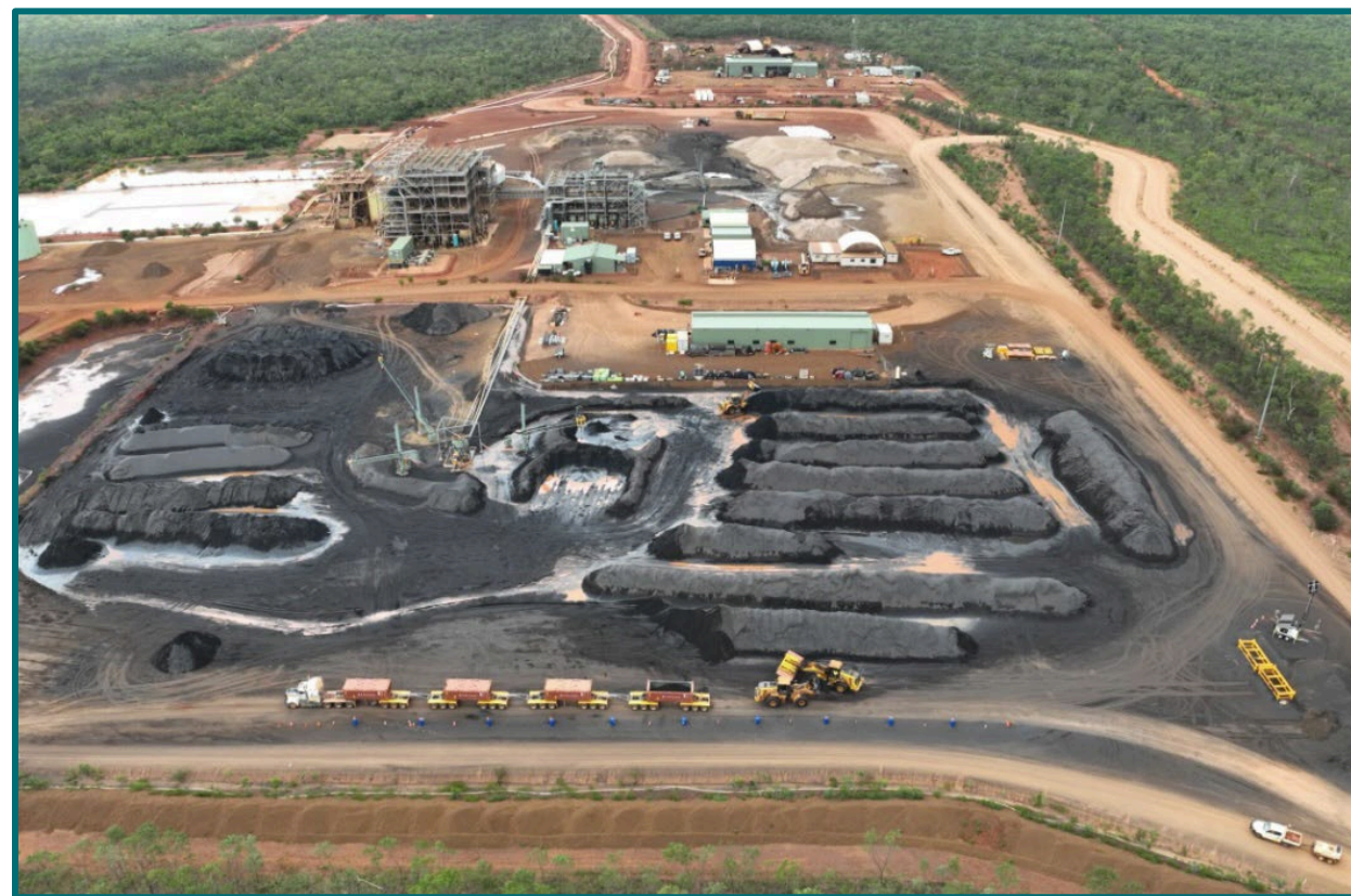
PROCESS PLANT AND PRODUCT STOCKPILES DECEMBER 2024
