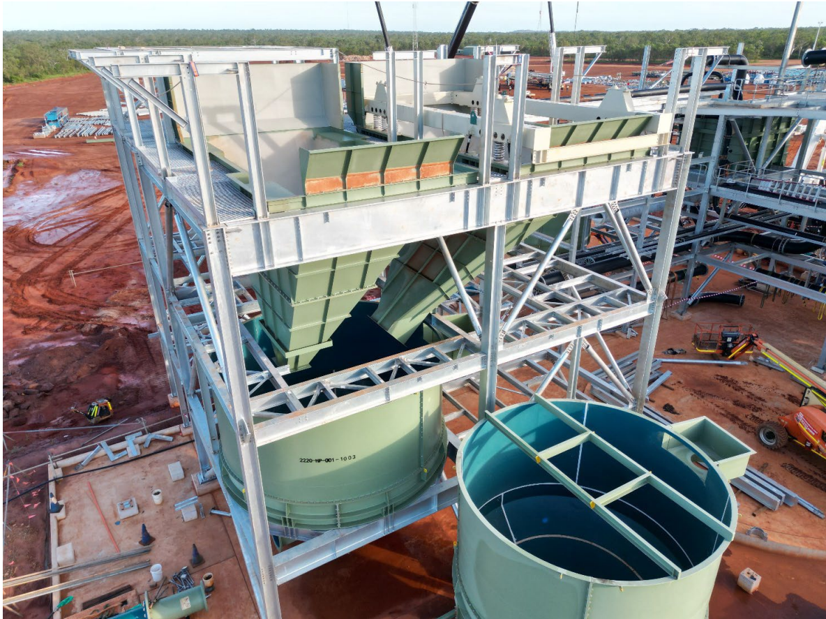
Image 4: Screen Building – installation & construction progress
