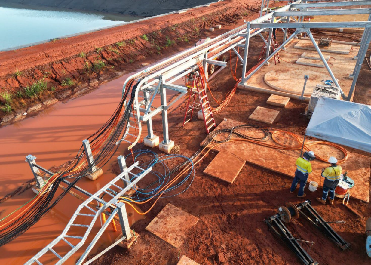
Image 8: Electrical cable installation
