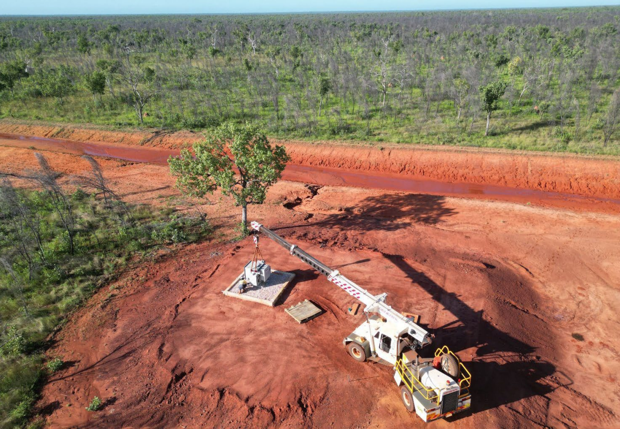
Image 7: Borefield Transformer installation
