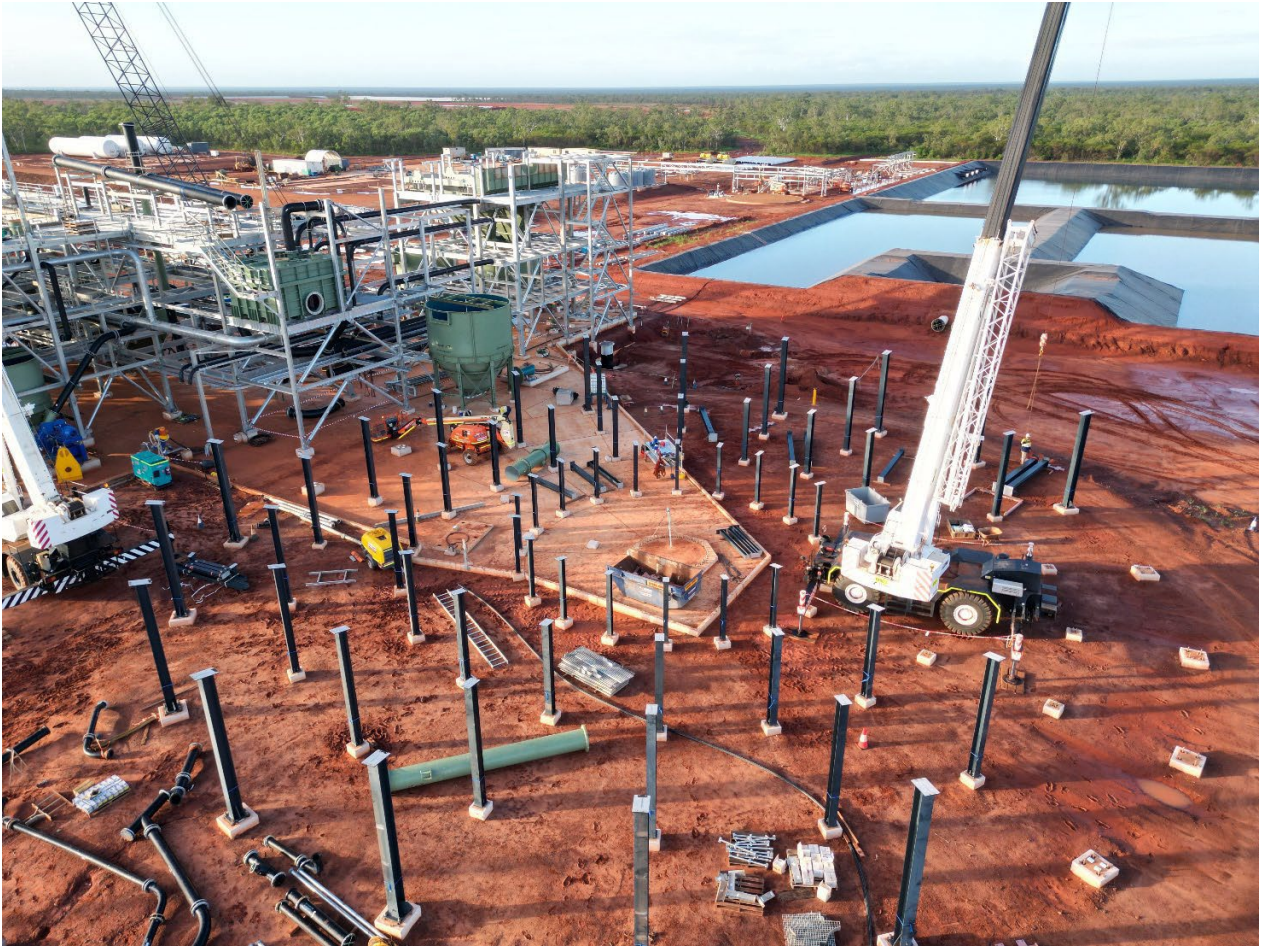
Image 9: Thickener Area – column installation
