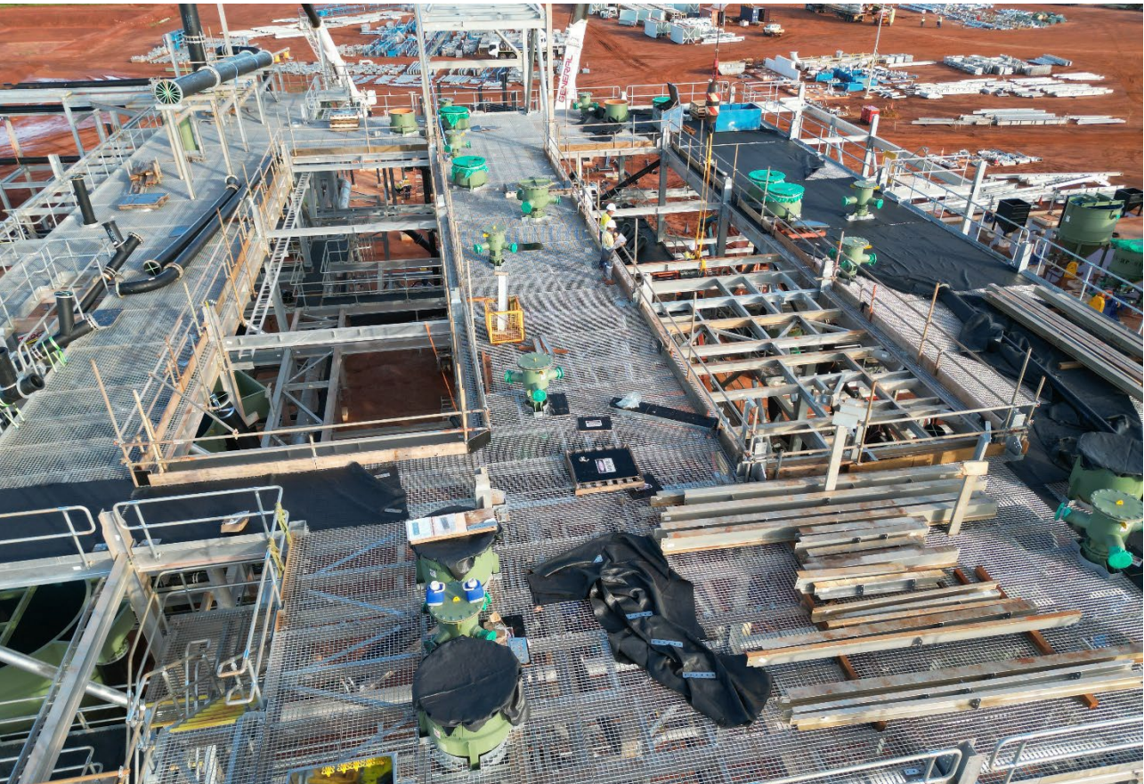
Image 3: Wet Concentrate Plant – construction progress
