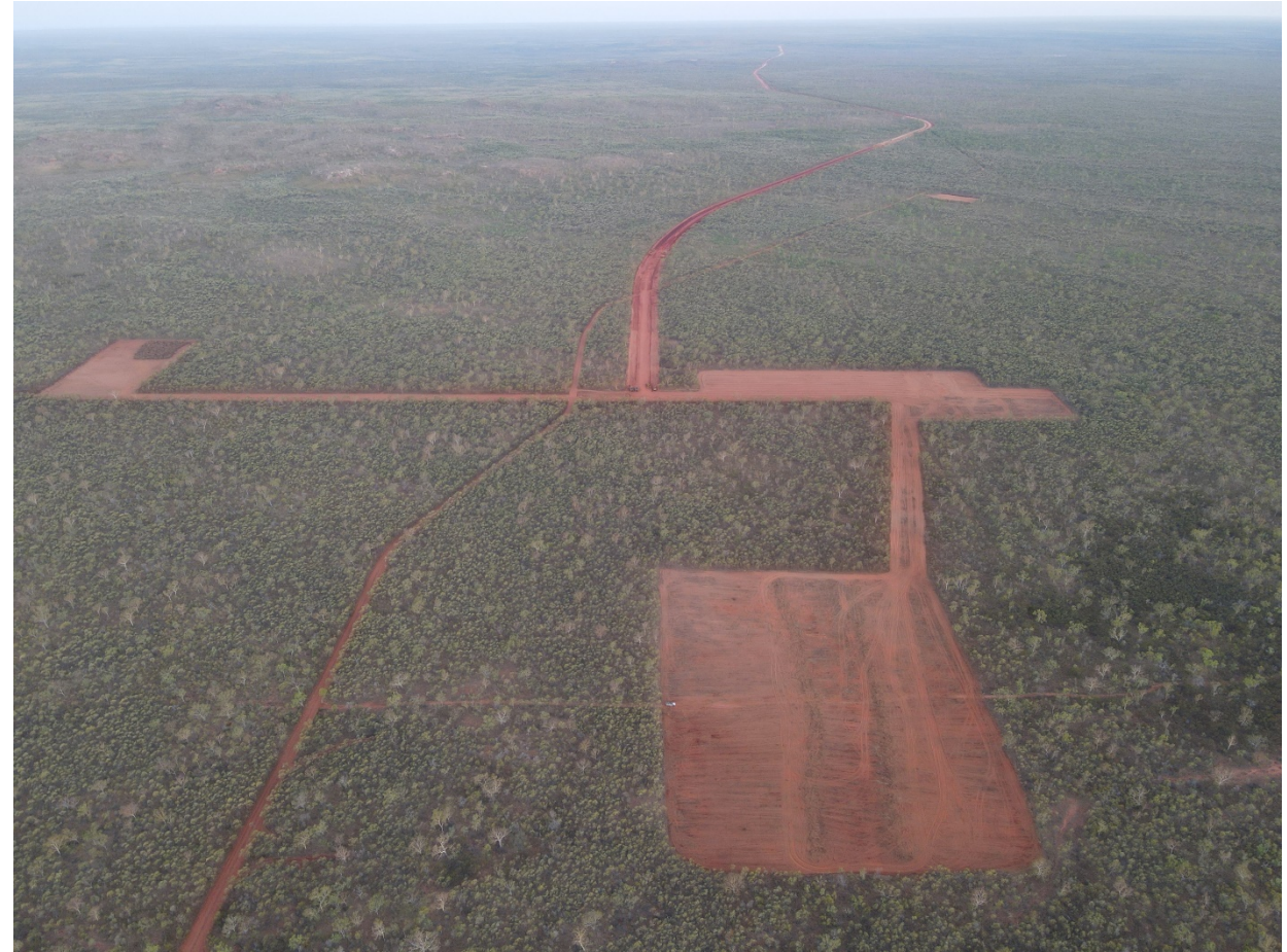
Aerial view of cleared process plant area and access road
