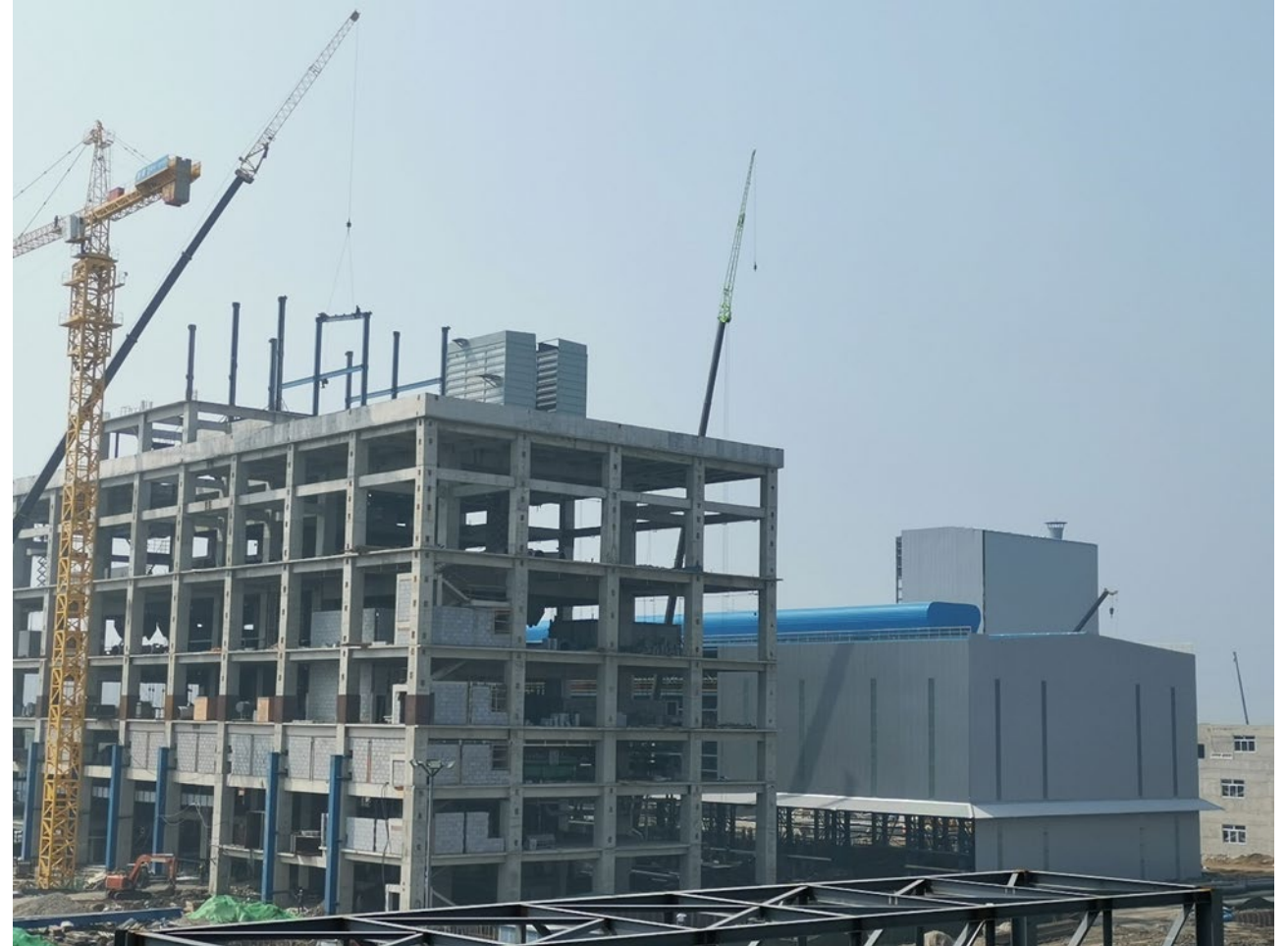
Yansteel Titanium Dioxide Plant under construction
