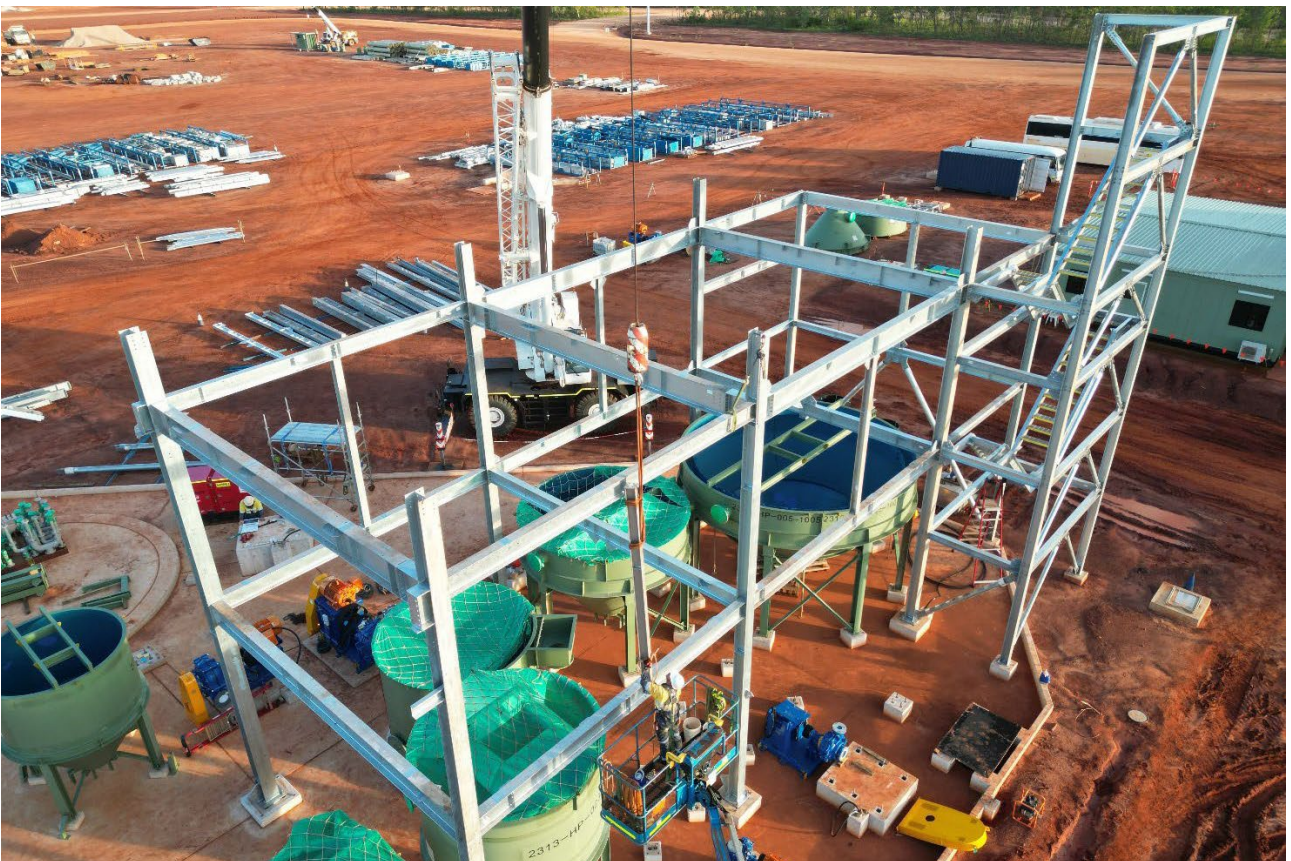
Image 3: Concentrate Upgrade Plant - steel installation
