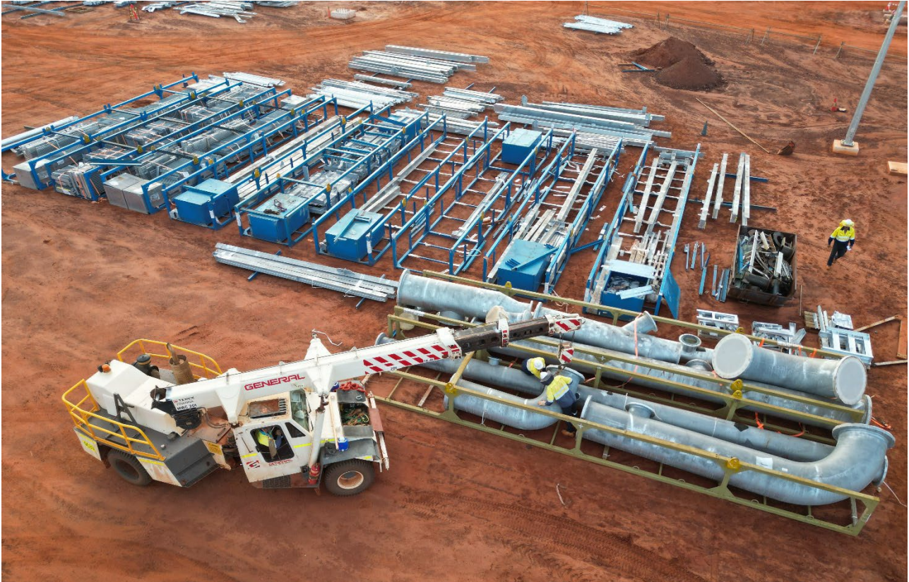
Image 6: Unpacking of steel piping and cradles at site laydown area
