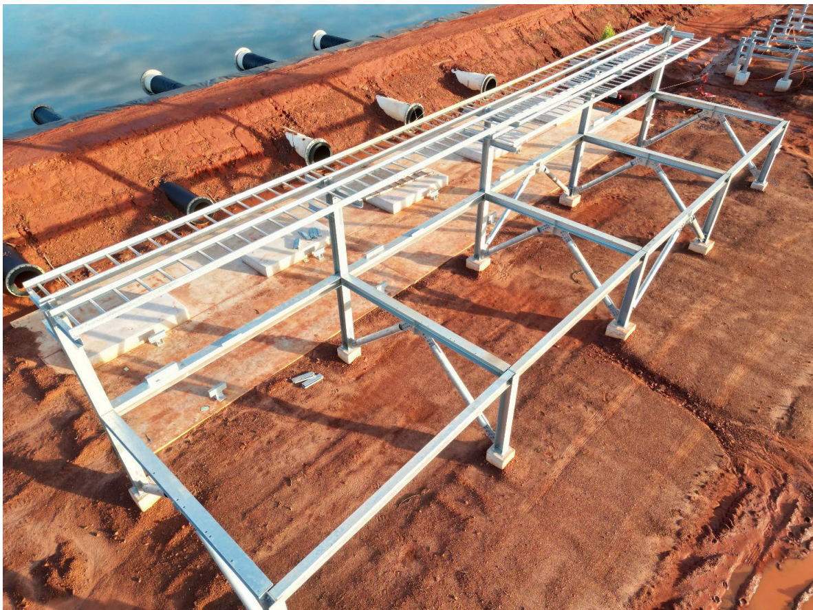
Image 5: Process Water Area framework & cable tray installation
