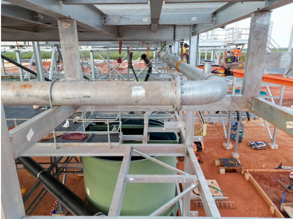
Image 4: Wet Concentrate Plant steel piping installation
