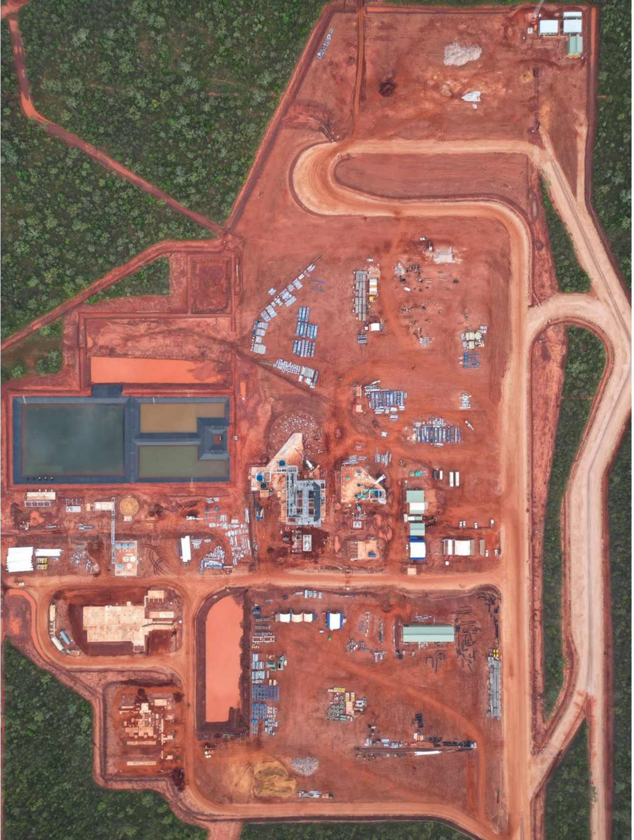
Image 1: Thunderbird Plant Site – aerial view (February 2023)
