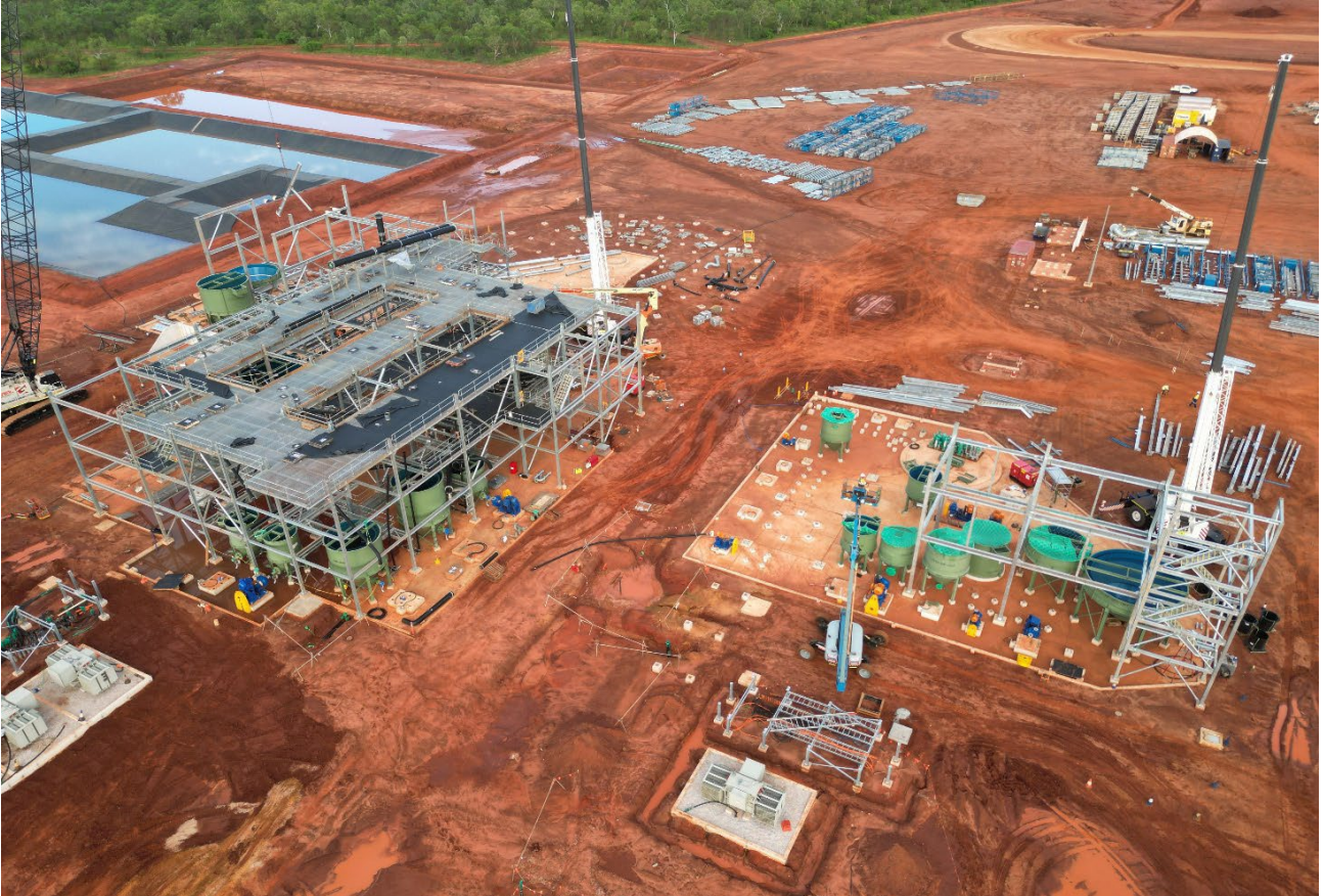
Image 2: Wet Concentrate Plant & Concentrate Upgrade Plant progress
