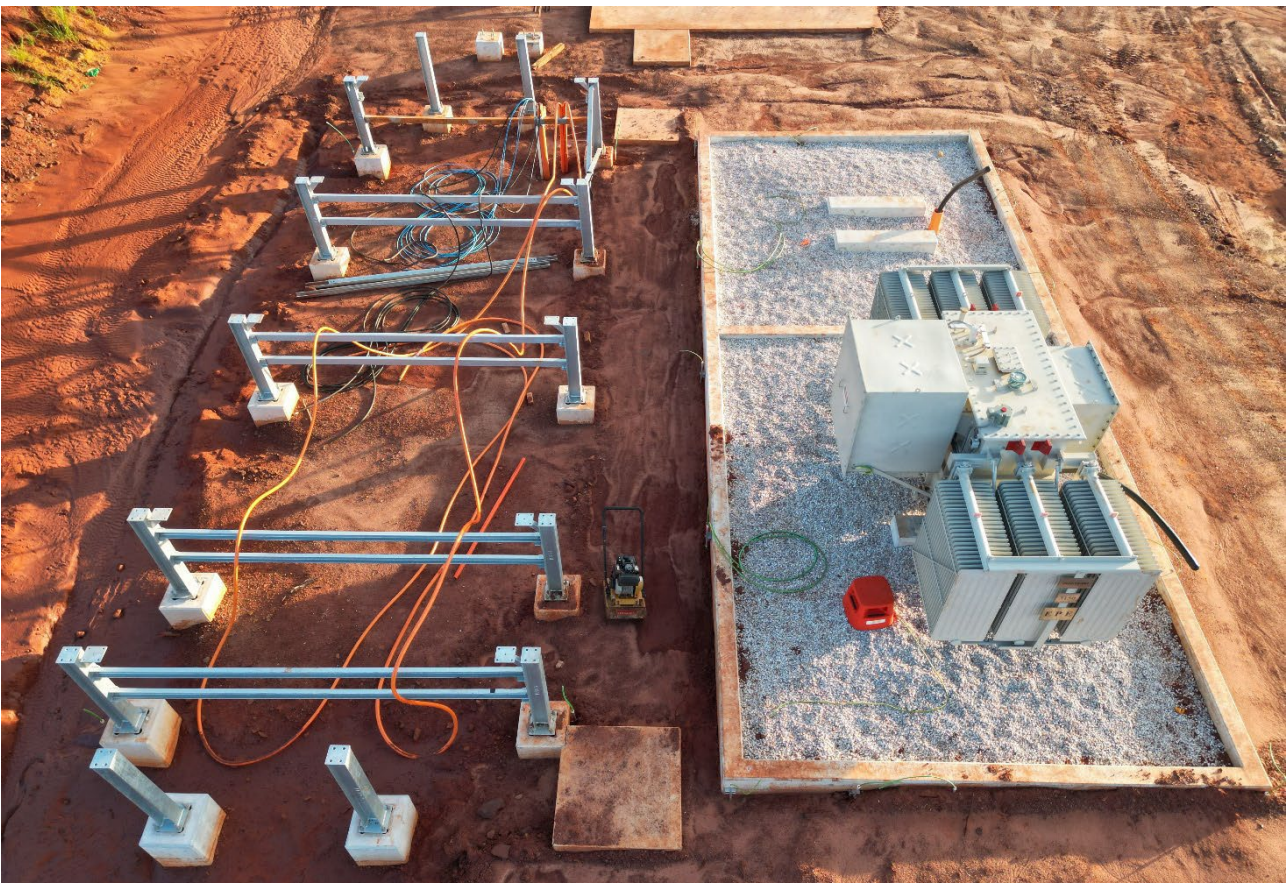
Image 7: Process Water Area sub-station – electrical works
