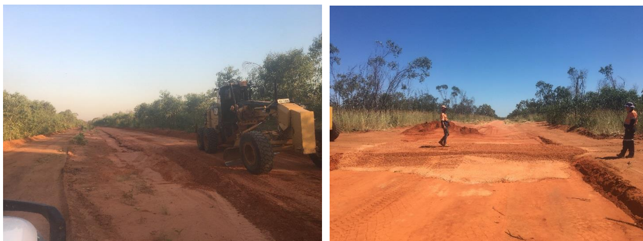
Figure 3 & 4: Upgrade of site access roads
