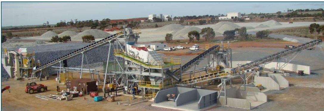
Luznac's Three Springs mine and new talc beneficiation plant. Source – Rio Tinto Minerals media release 16 November 2010
