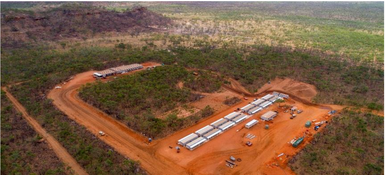
Figure 4: (above) Construction Ready Thunderbird accommodation village
