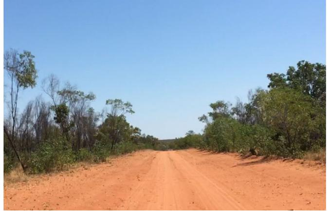
Above: The ~30km unsealed Thunderbird access road is pretty well established. The first 19km will be used and a new ~11km dual lane unsealed road will be constructed, suitable for quad trailer road trains up to 53.5m long.
