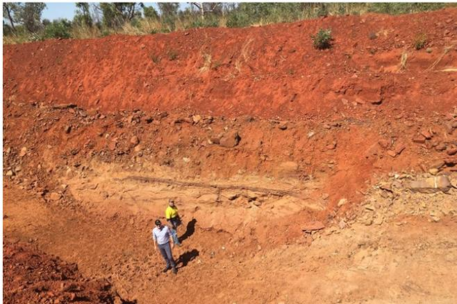
Above: Standing in one of the three test pits. This pit was excavated with a D10 dozer.
