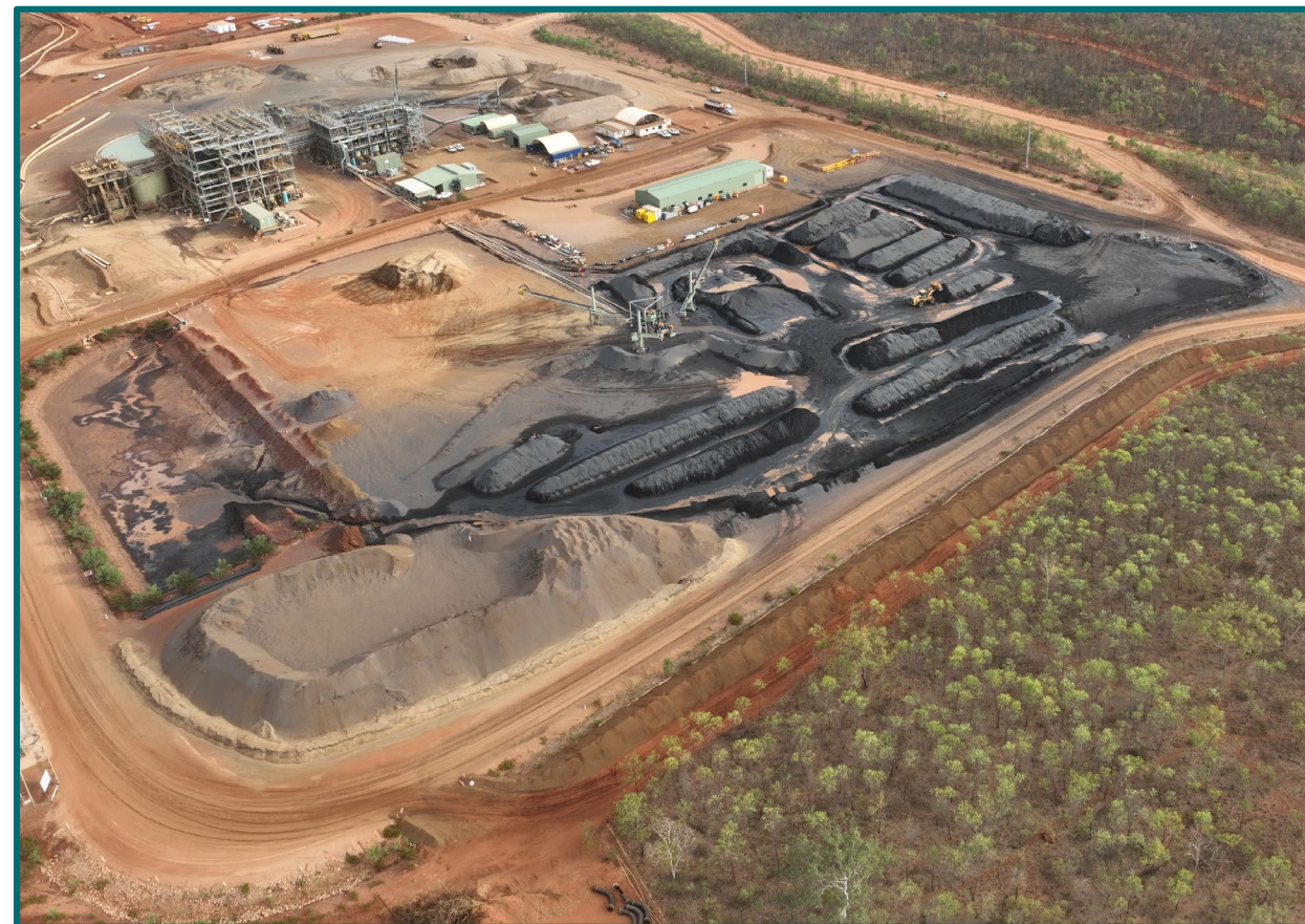
PROCESS PLANT AND PRODUCT STOCKPILES SEPTEMBER 2024
