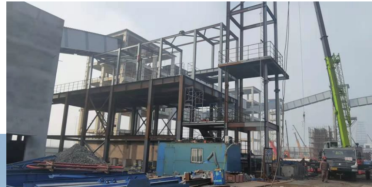
Magnetic separation plant construction activities
