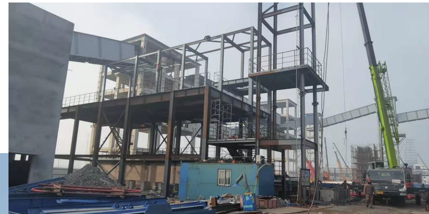
Magnetic separation plant construction activities
